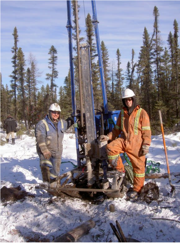
Shawn Bishop, driller, and Scott Kingdon, helper, pose with the portable drill rig. The five-foot length of hollow-stem auger is being lowered into the bore hole.
